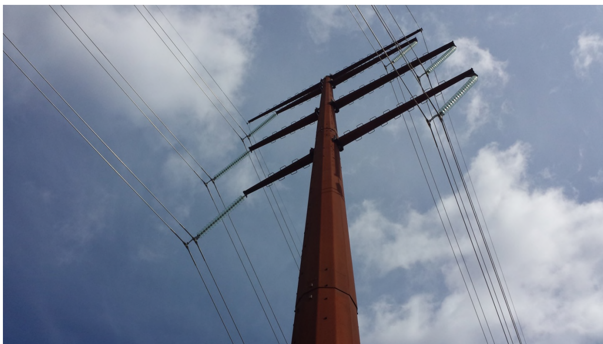
Fig. 1 – A 150 foot tall 345 KV power pole
