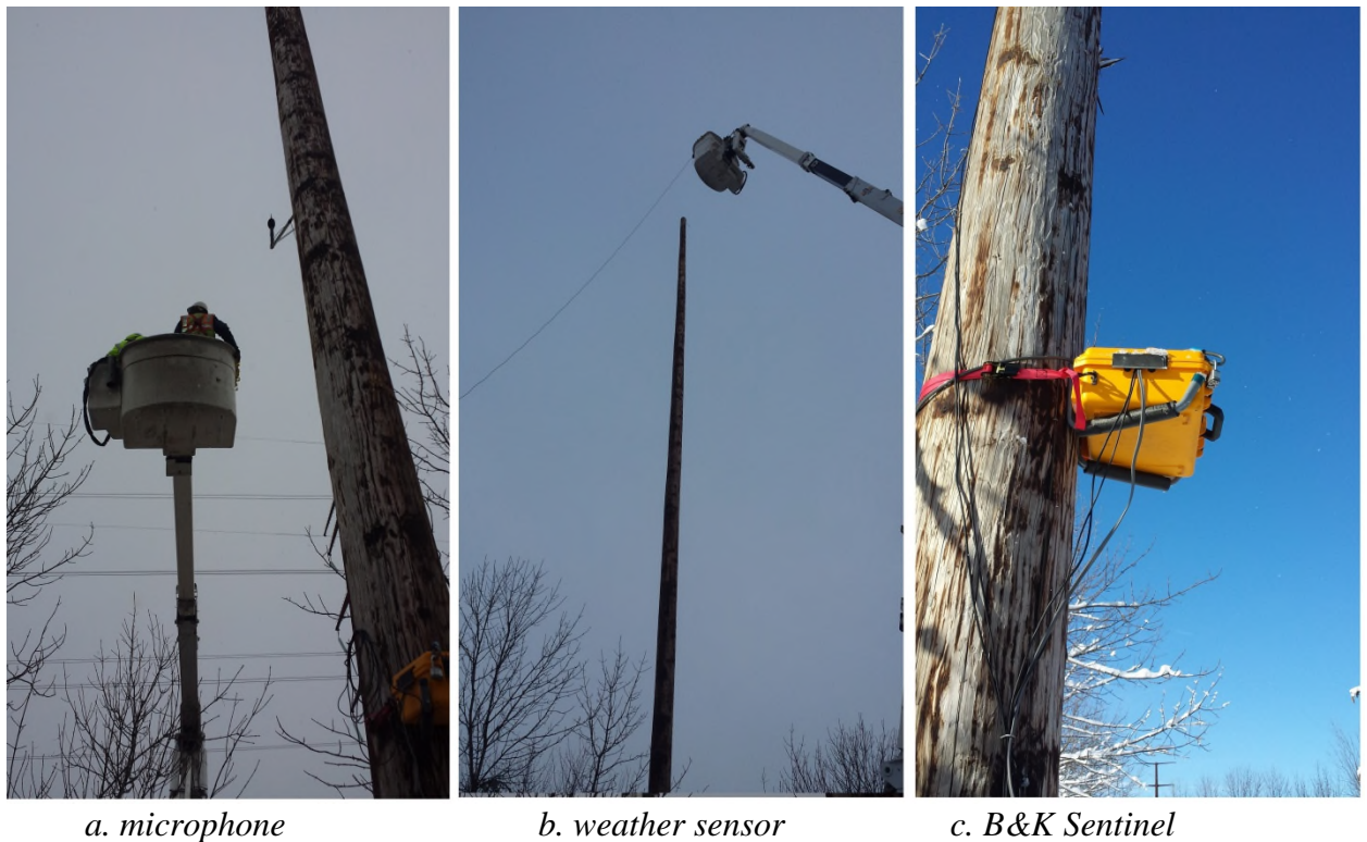
Fig. 2 – Installation of the sound monitoring and weather instrumentation
